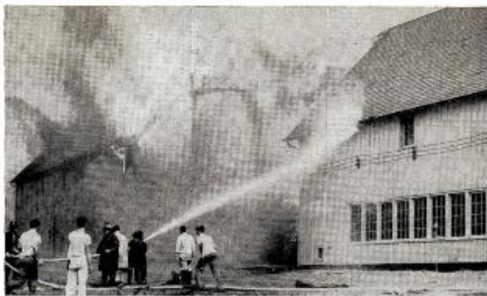
Flames eat close to the WVCH transmitter building.
